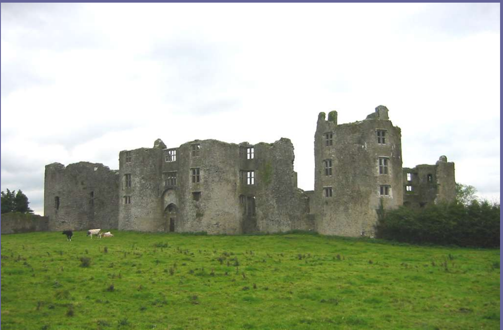
Roscommon Castle from the north east showing the twin-towered gatehouse
